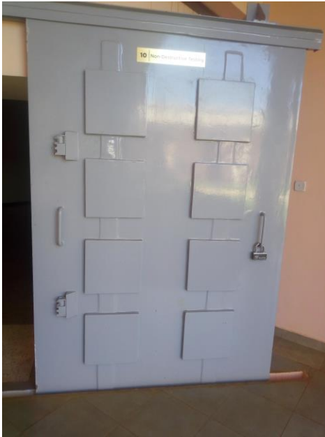
TEMDO radiation protection doors installed at Tanzania Atomic Energy Commission laboratories.
